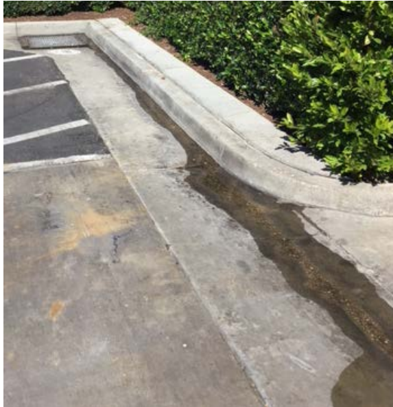
Illegal non-stormwater discharge from a facility using a hose to wash the sidewalk.
