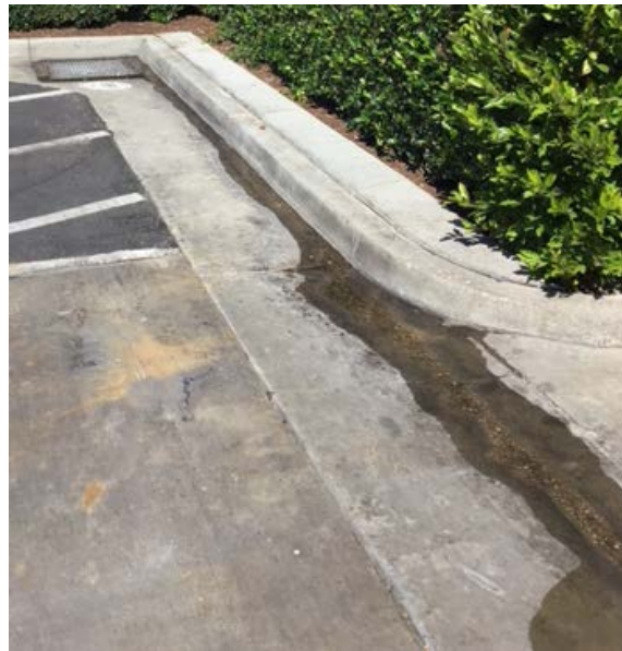
Illegal non-stormwater discharge from a facility using a hose to wash the sidewalk.
