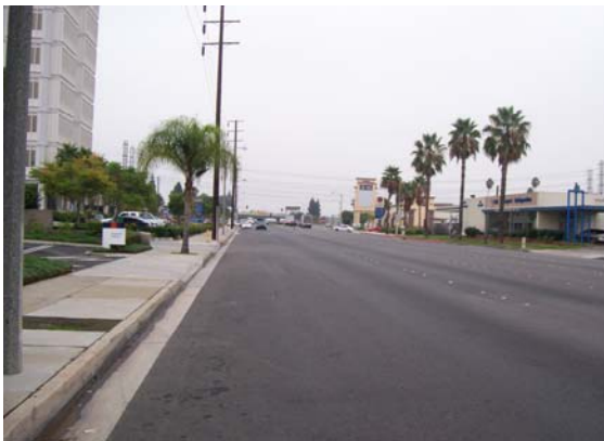
Washington Boulevard has undergone major improvements with more to follow.
