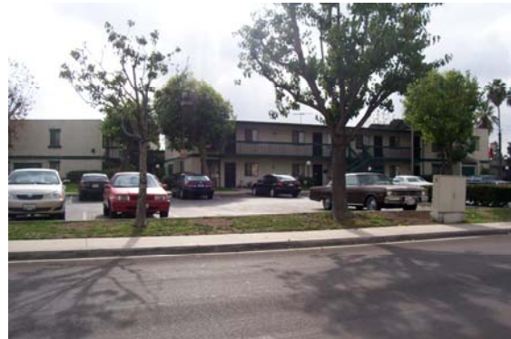
In spite of the city's small size, it has participated in the development of a number of senior housing projects.
