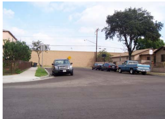
Caltrans recently completed construction of sound walls along the I-5 Freeway.
