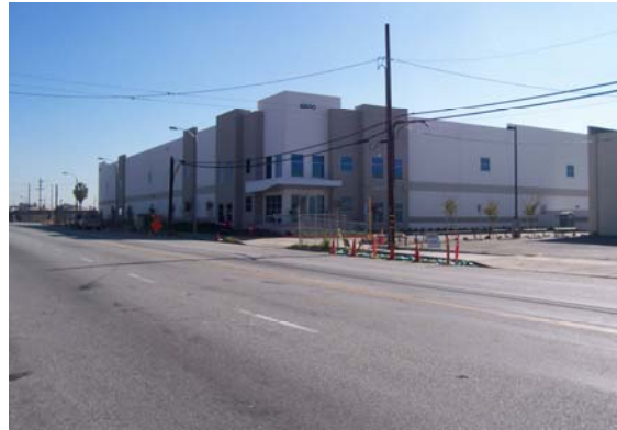
Industrial land uses are the dominant land use accounting for more than 60% of the city's total. This new development is located along Bandini Boulevard.
