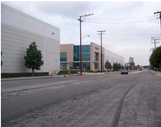
Newer light industrial buildings located along Smithway Street.
