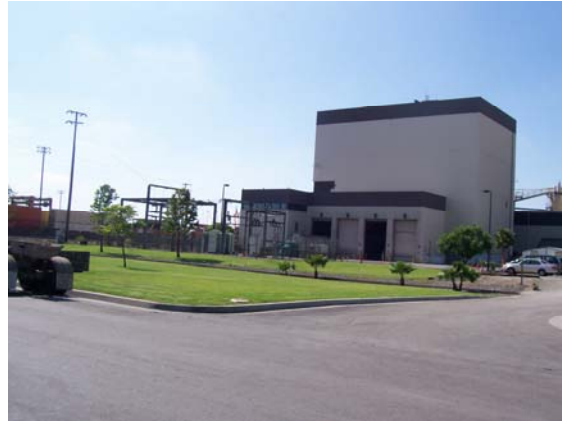
The Commerce Waste to Energy Plant has undergone continuous retrofits to decrease stationary emissions.
